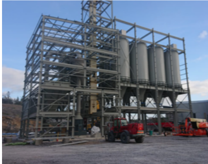
State of the art milling, classifying and screening plant for the simultaneous production of limestone filler and grits, supplied with a fully automated control system enabling 24/7 unmanned production
