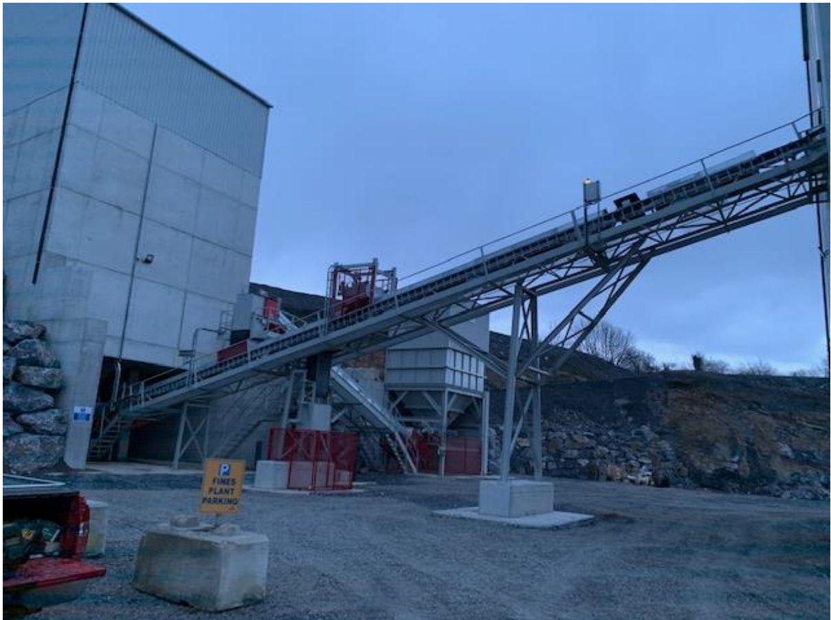
Primary and Secondary Feed Bunkers with Main Conveyor
