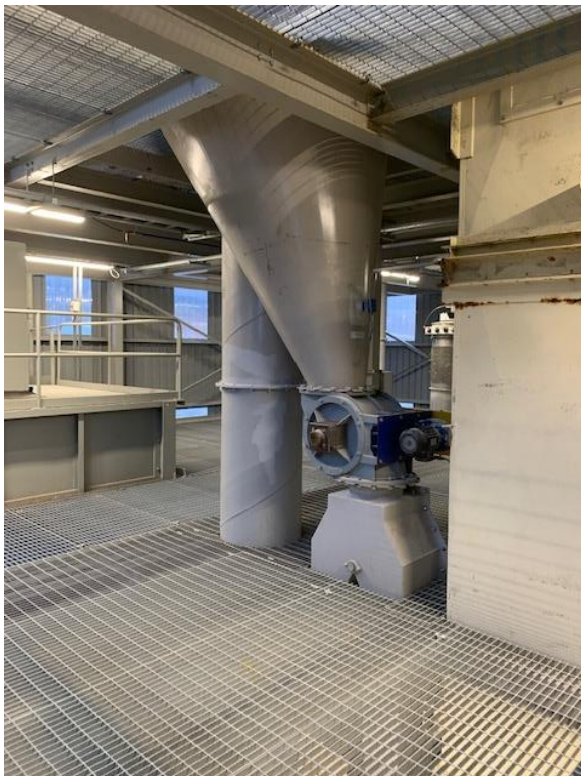
Classifier Rejects off-set cone with positional diverter valve allowing for regrind or transport via elevator to grits plant
