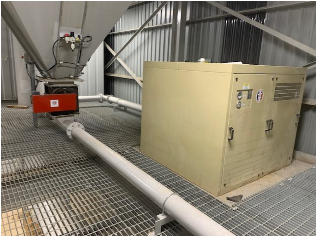
Blower and Surge hopper for product transfer to silos
